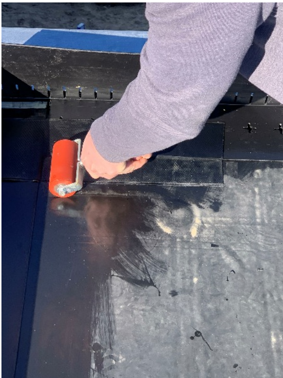
REMOVE PAPER COVER, SMALL SECTION AT A TIME AND PRESS EDGING INTO SEAM TAPE
