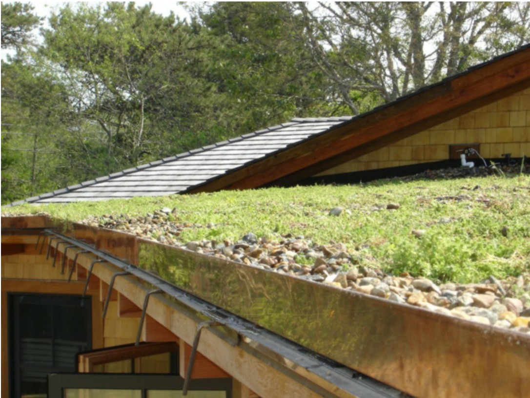
SPECIALTY EDGE DETAIL, COPPER WRAP (SHOWN HERE)
