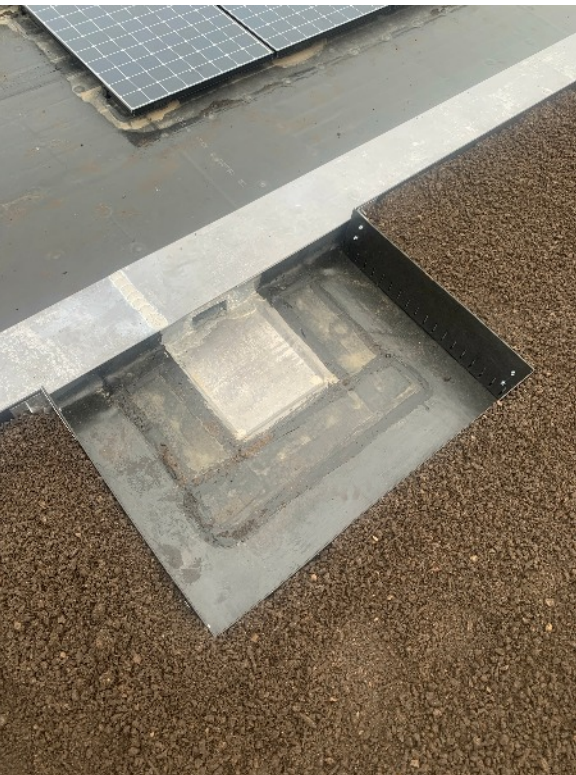
SECURE CORNERS WITH GLTI METAL CORNER BRACKETS
