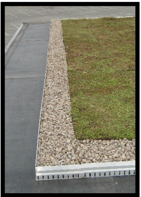
3/4 clean stone as ballast edge Or pavers *Option pending detail
