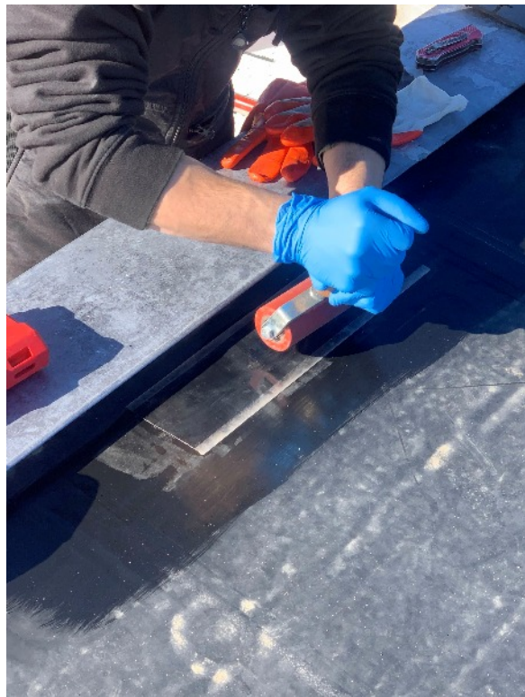
PRESS DOUBLE SIDED SEAM TAPE INTO WATERPROOFING
