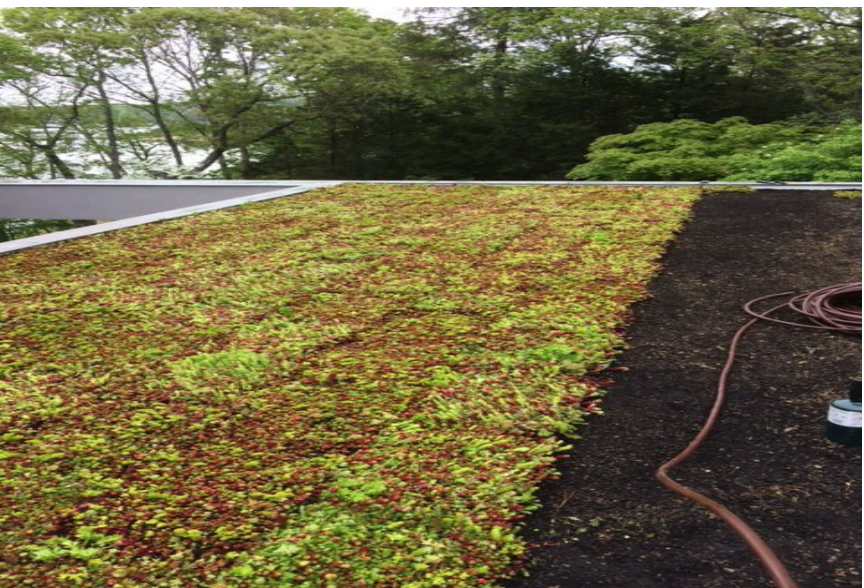
Install Irrigation Under Mats
