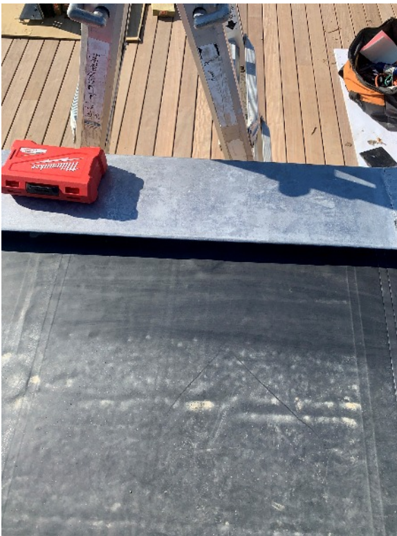
CLEAN / PRIME WATERPROOFING AND EDGING
