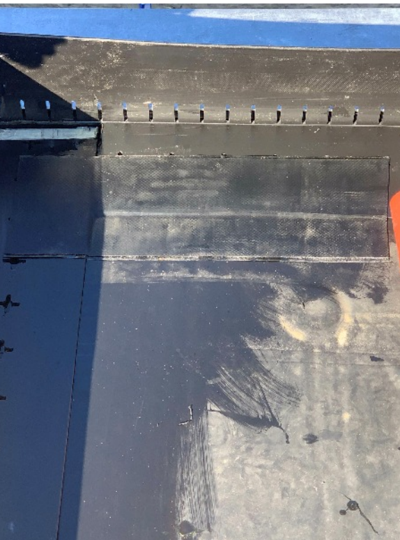
ROLL SEAM TAPE FOR SECURE BONDING
